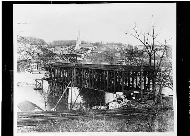
The 1895 Falls Bridge under construction, East Falls in the distance.
