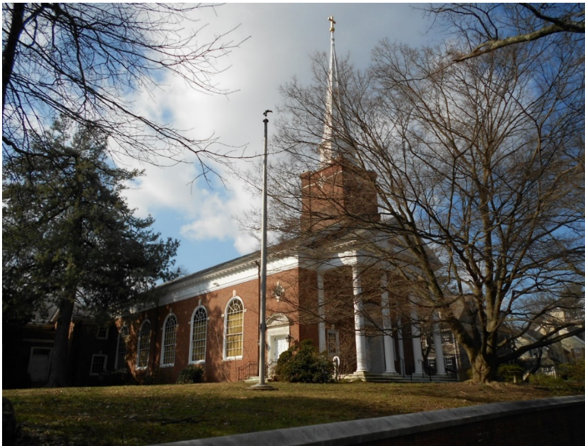
Figure 9: 3/4 view of church looking west. Nancy Pontone, January 2019.
