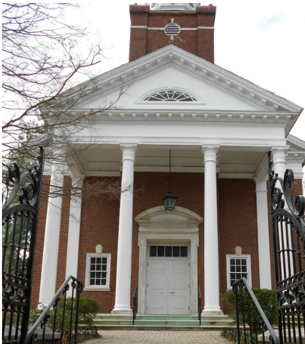
Figure 11: Front elevation of church looking southwest. Nancy Pontone, March 2019.
