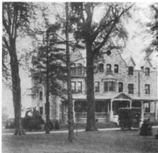
Ravenhill residence of Mrs. E. Courtland Penfield, daughter of Wm. Weightman, on the site of the former residence of Mr. Weightman. From the C.K. Mills Collection.
