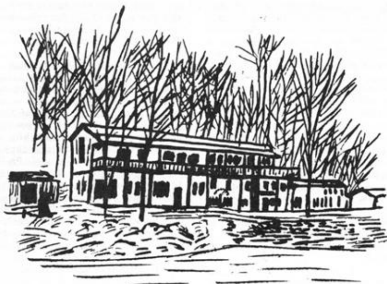
The Old Log Cabin on Wissahickon Drive
