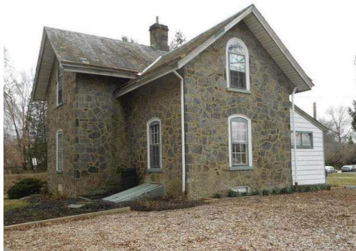
Figure 10- 3/4 northeast facing view 3001 W Coulter Street. Nancy Pontone, February 2020.
