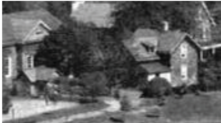
Figure 5 – 1938 photo northwest facing view of subject property, https://www.penncharter.com/uploaded/Yearbook_Archives/1930s/1938.pdf
