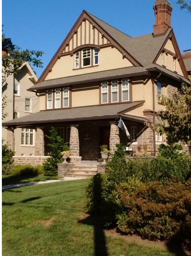
Figure 20: Midvale Avenue at Fox Street. Tudor Revival and Arts and Crafts Style. From 1907, it was one of the first built by the developers and was used in an early advertisement. Architect not determined. Steven Peitzman, August 2019.
