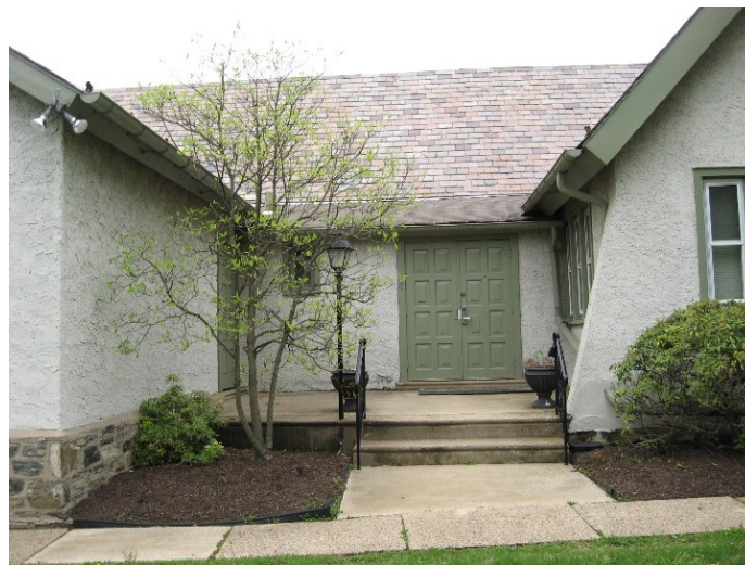
Figure 13: West view of 1938 addition. Steven Peitzman, June 2019.
