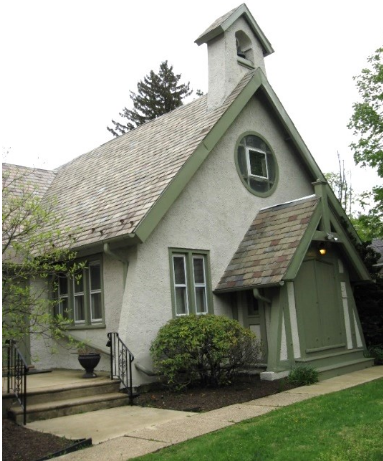
Figure 9: 3/4 view of chapel at 3625 McMichael Street, facing south east. Steven Peitzman, June 2019.
