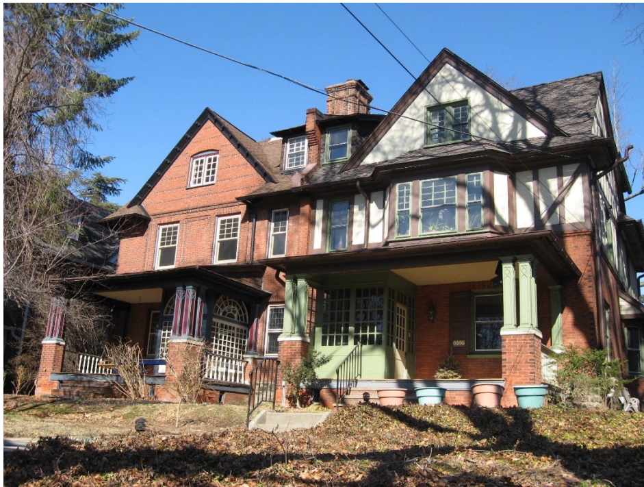
Figure 22: Twin houses on the 3000 block of Queen Lane. Architect not determined
