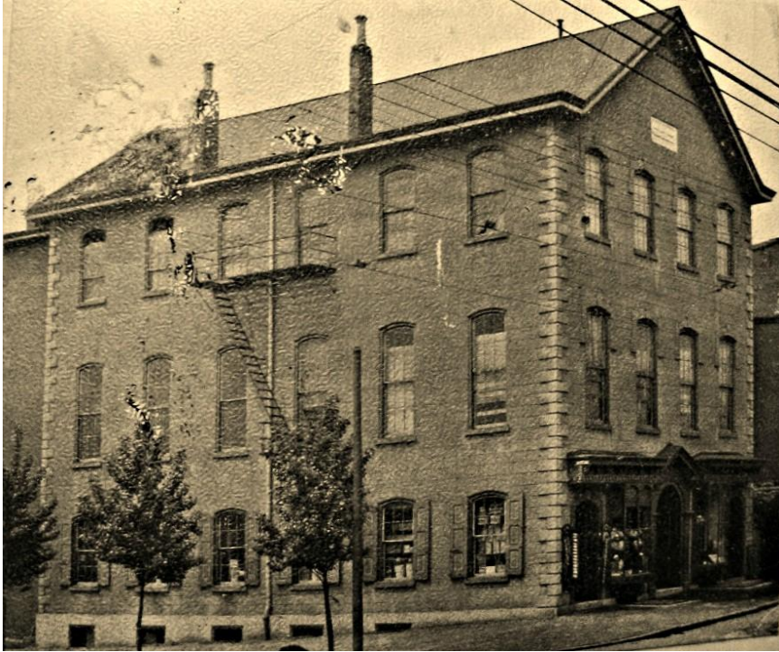
Figure 5: A c.1900 photograph of Odd Fellows' Hall shows an early configuration of the storefront. It also shows exposed quoins and a stone panel inset below the peak of the roof. Source: Historical Society of Pennsylvania, Chadwick Collection (Collection 1844), "Pictures: Falls of Schuylkill. No. 3."
