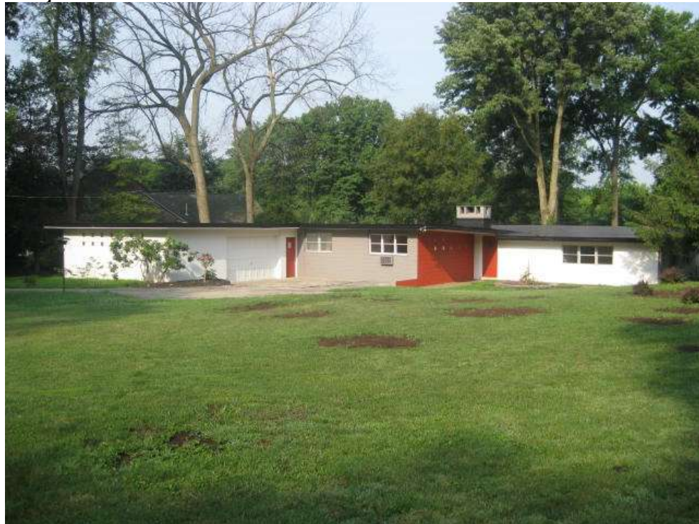
1951-1974-2009 South Elevation Before -Roofline showing original 1951 vents from toilet room and darkroom. 1974 Rolled Asphalt Roof with Aluminum silicate coating is in place.
