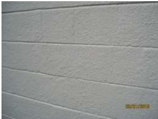
1951- Cinder block with parging and scored joints
