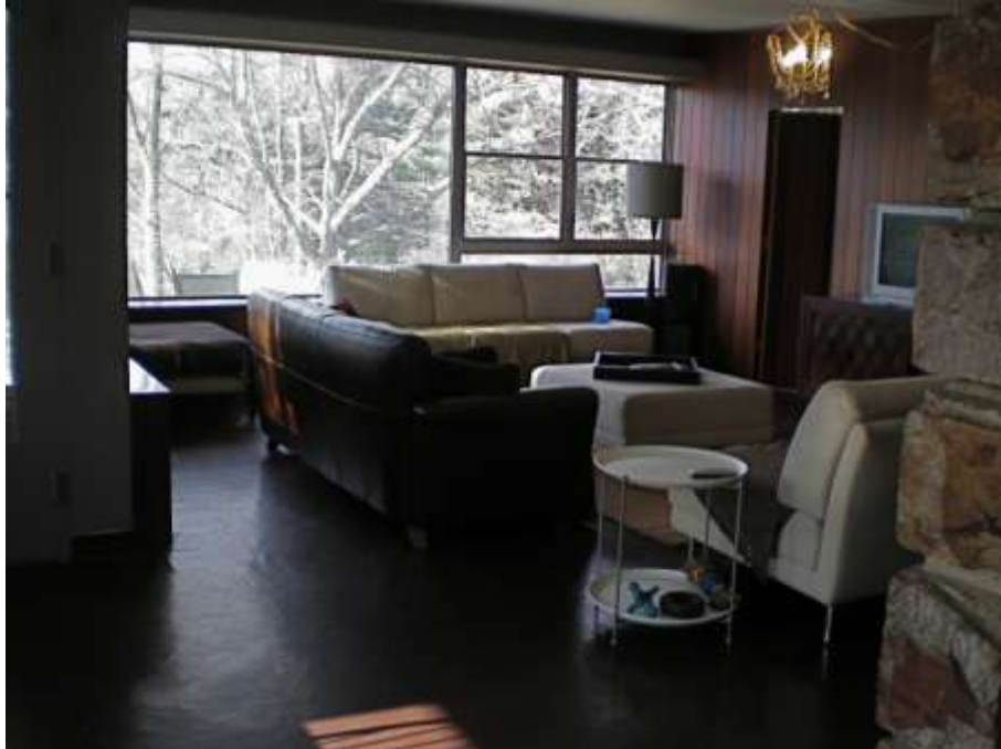
1951 Living Room showing 9x9 brown vinyl asbestos tiles, mahogany paneling
