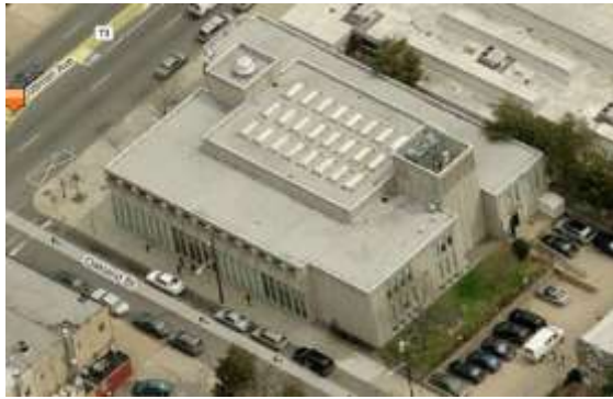
District Health Center #10
