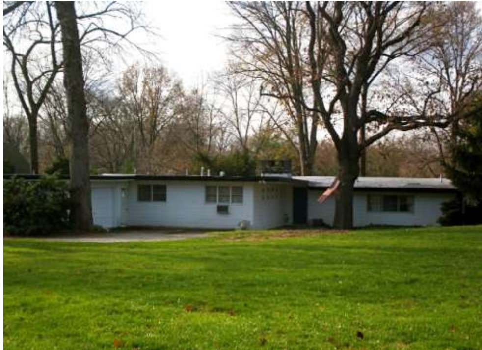
1951-1974-2009 South Elevation Before -Roofline showing original 1951 vents from toilet room and darkroom. 1974 Rolled Asphalt Roof with Aluminum silicate coating is in place.
