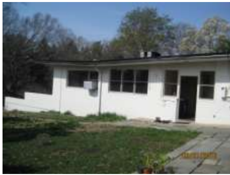
Butterfly Roof at 3419 W. School House Lane
