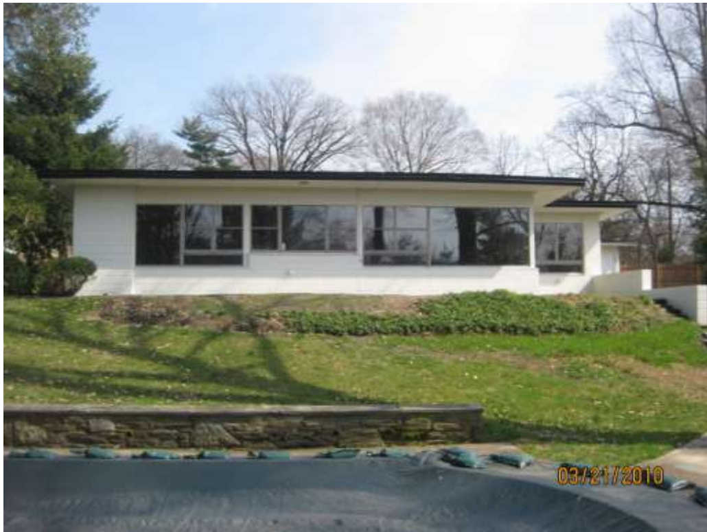
1951-West Elevation showing ribbon windows
