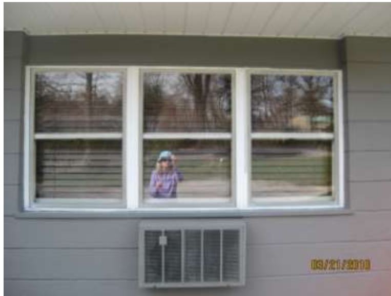
1974-Double Hung Aluminum windows with plywood panel above
