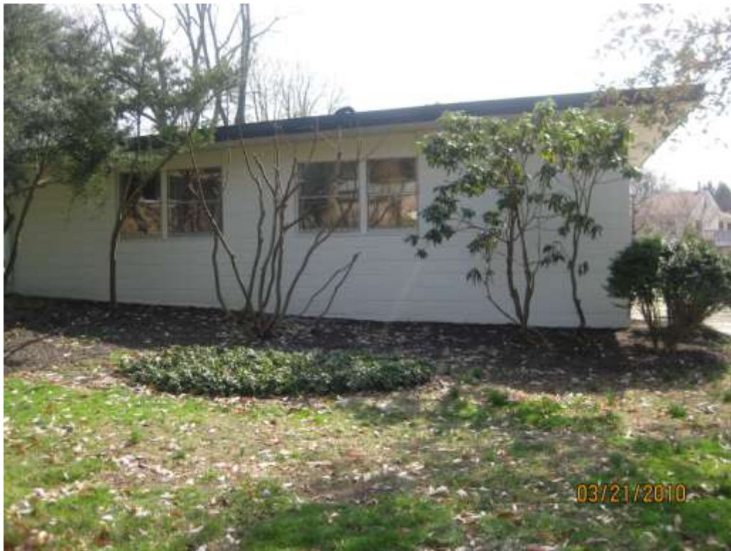
1951 -North Elevation showing punched windows
