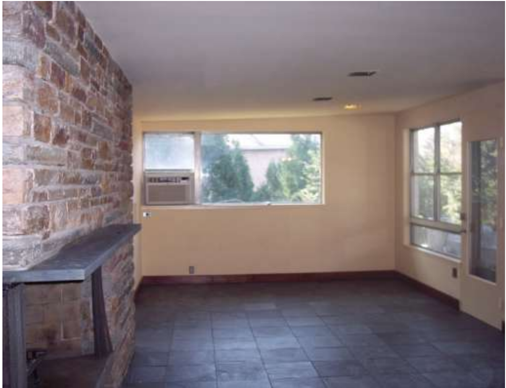
2009 Living Room Dining Room showing slate floors, texture of slate replicates texture of original vinyl asbestos tile. Color of slate matches mantle.
