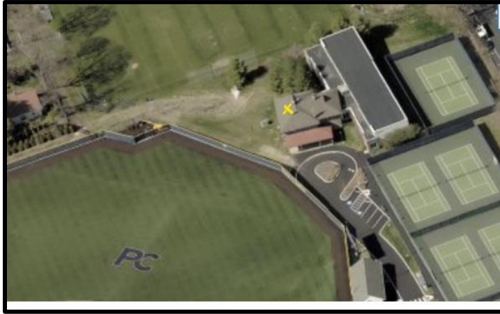
Figure 3: Location of building (x) on north campus of Penn Charter
