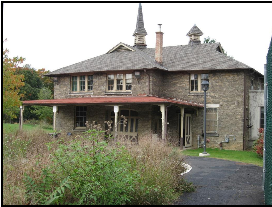
Figure 5: The Stable and Carriage House looking north to the front. All current photos are by the nominator.
